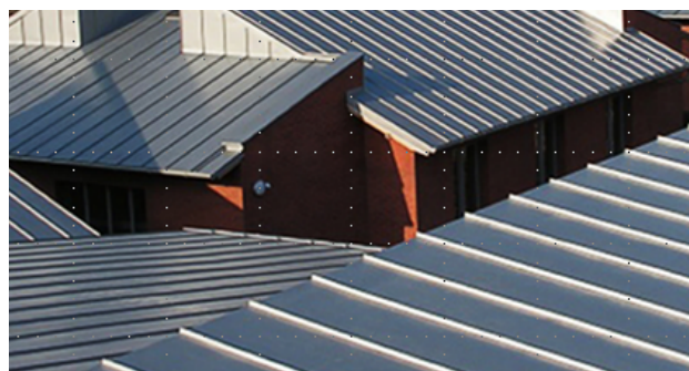
Standing seam roof and rainwater systems ©Lindab & Liberty Dudelange
